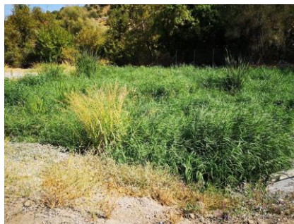
Figure 2. Saturated vertical flow constructed wetland (VF SAT)
