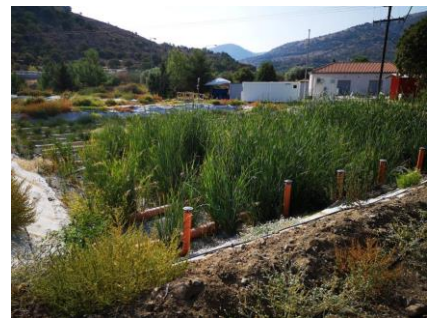
Figure 3. Unsaturated vertical flow constructed wetland (VF UNSAT)
