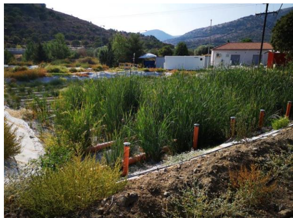
Figure 3. Unsaturated vertical flow constructed wetland (VF UNSAT)
