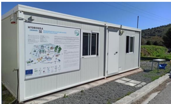
Figure 4. In situ control room
