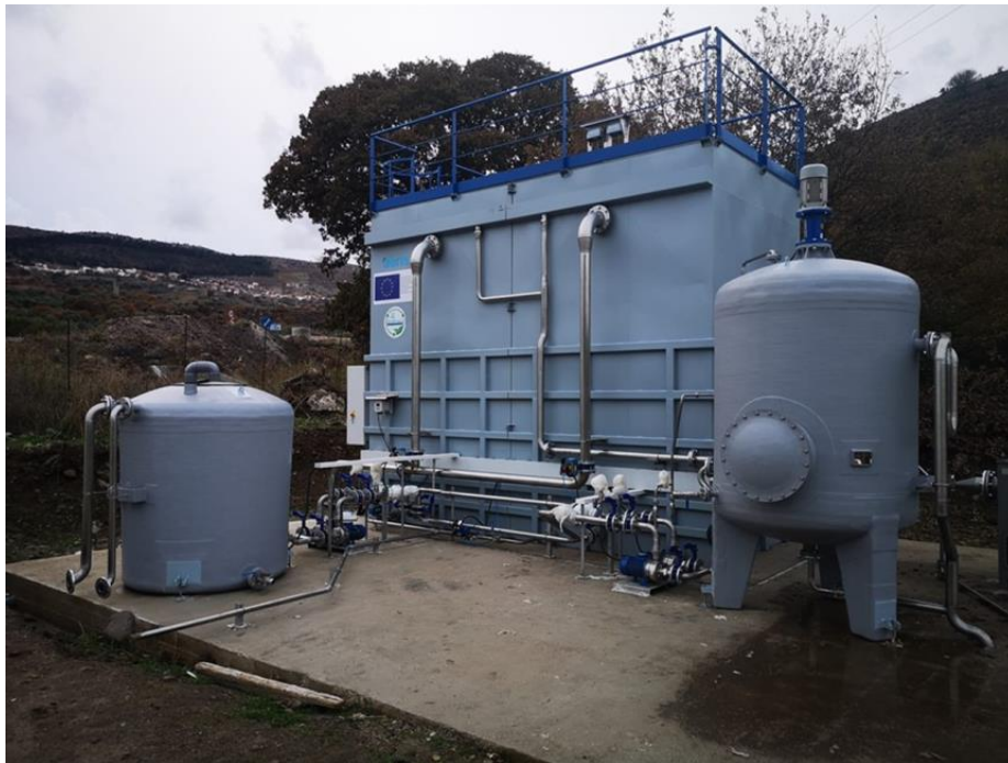
Figure 1. Anaerobic reactor (AR)
